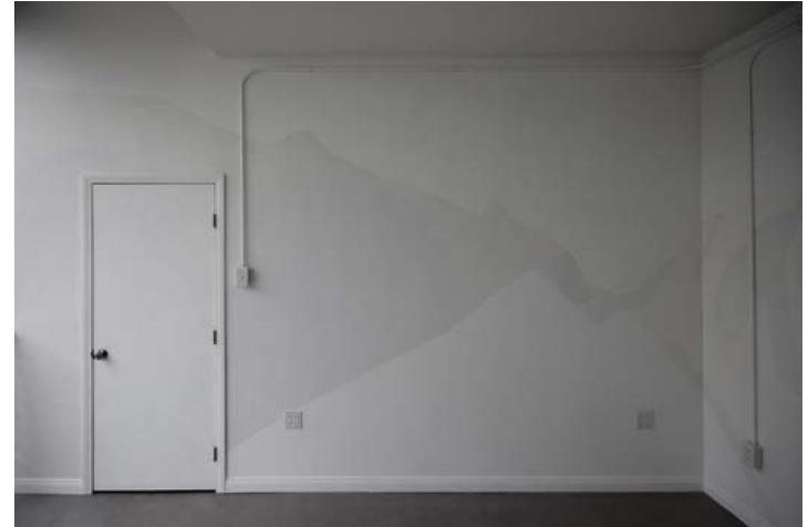
Old wall with mountain panorama, molding and conduit.
